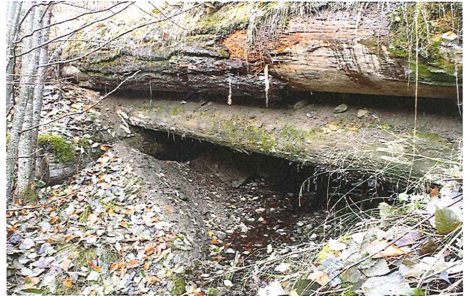
CK2007 From Downstream
