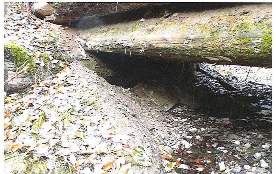
CK2007 Right Abutment
