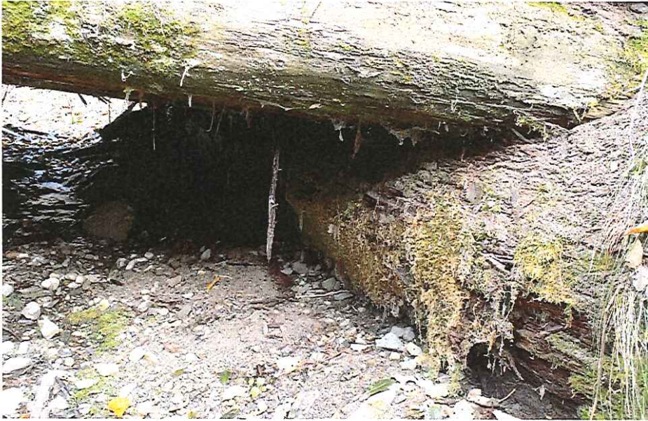
CK2007 Left Abutment
